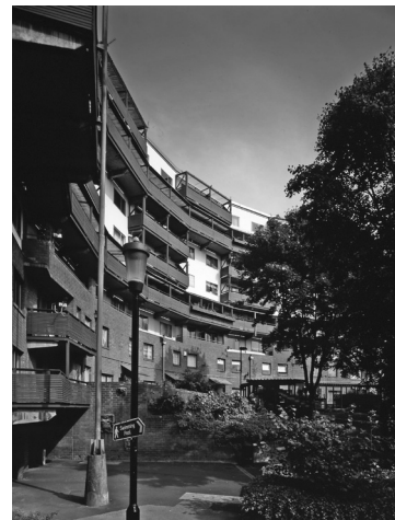
8 The wall of the Byker Estate
